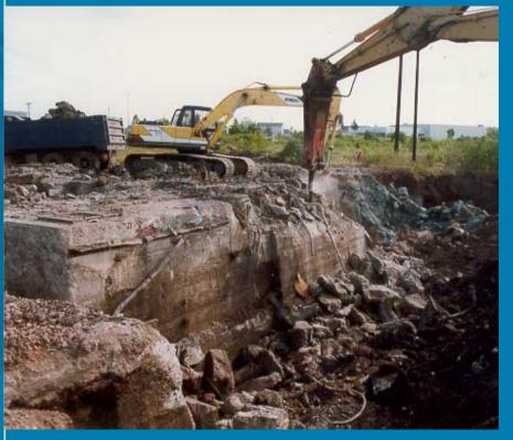
Reused 60,000 tonnes of concrete on site as base and drainage levels for roadw ays and playing fields
